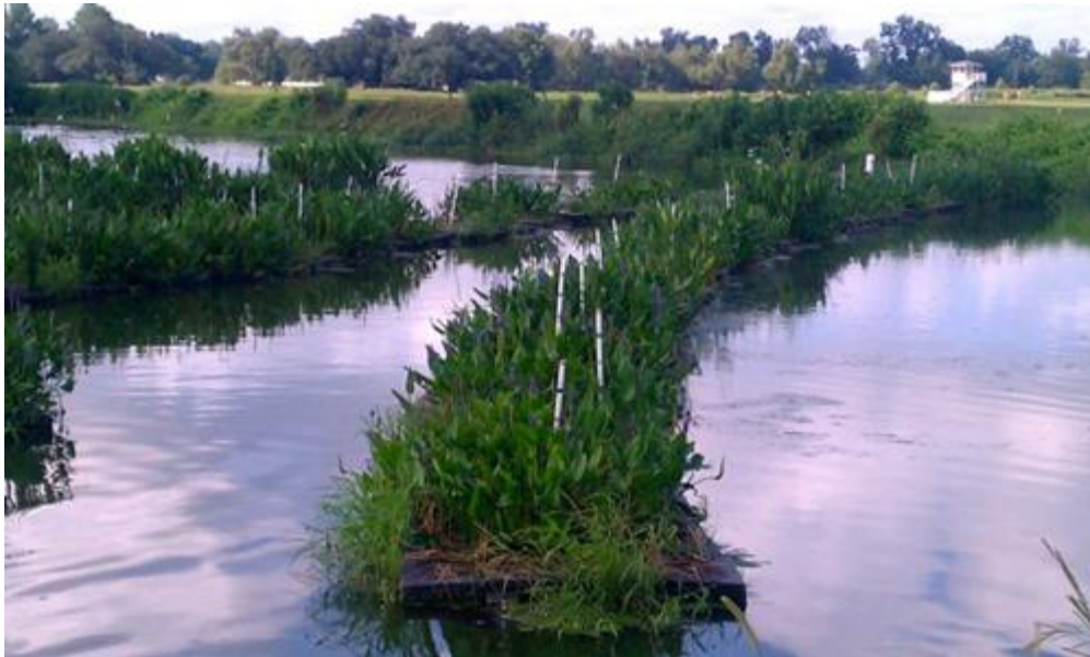
Slika 5: Primer plavajočega čistilnega otoka v Elayn Hunt Correctional in St. Gabriel, Louisiana. Vir: http://www.wateronline.com/doc/wastewater-pond-uses-floating-wetlands-for-nutrient-removal-0001 , 22. 1. 2017
